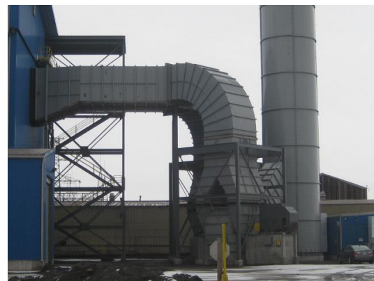
Multiple I.D. Fan Arrangement w/Access & Support
