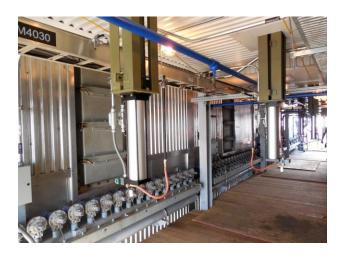
Bag installation is a snap with tool-less double bead snap band installation into the cell plate.
